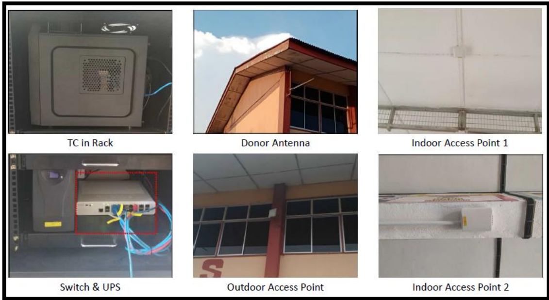
Figure 7 shows the installation of Hardware devices at the school.
